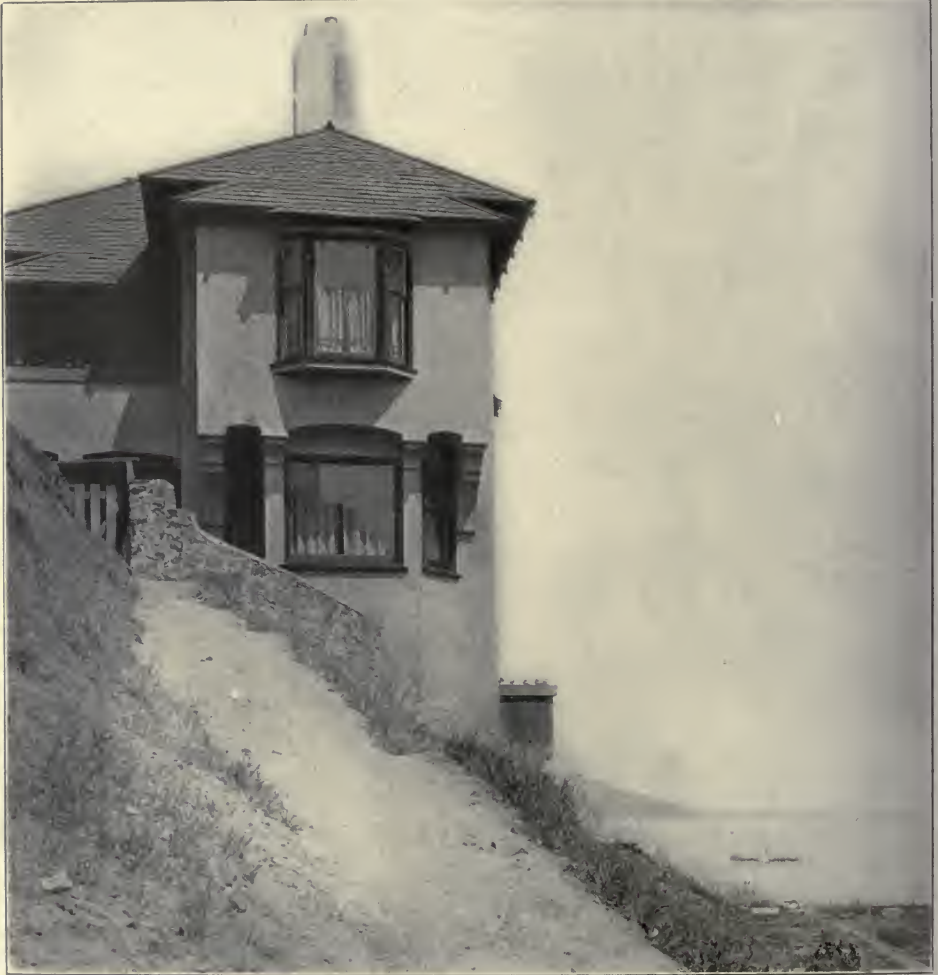
FIG. 2. THE SOUTH END OF THE DWELLING, SHOWING THE ROUGH TRAIL LEADING UP VALLEJO ST. TO THE SIDE DOOR—THE HOUSE OF MR. LIVINGSTON JENKS.
