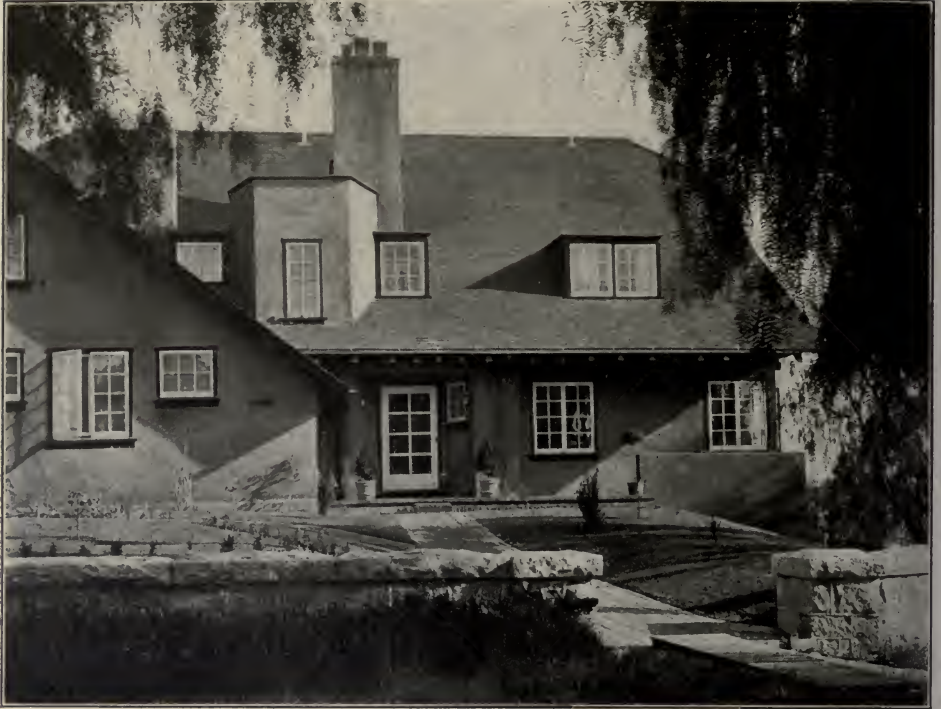
THE COCHRAN HOUSE.
