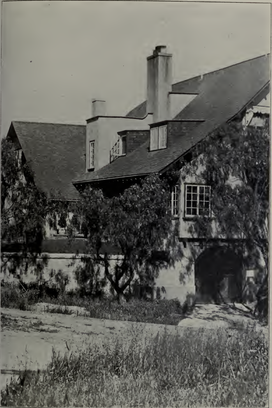
THE COCHRAN HOUSE.
