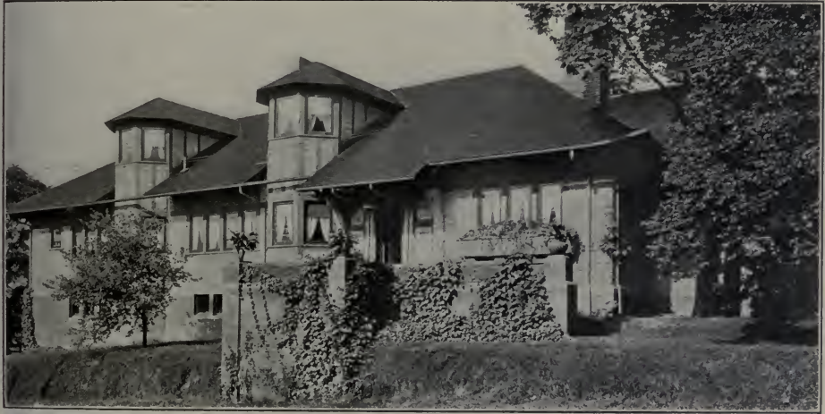
FIG. 1. MRS. WATERMAN'S HOUSE AT PARKERSBURG, WEST VIRGINIA.
