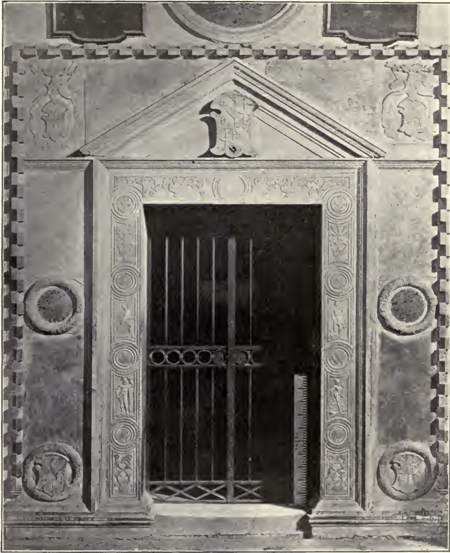
FIG. 9.—AN INTERIOR DOORWAY.
