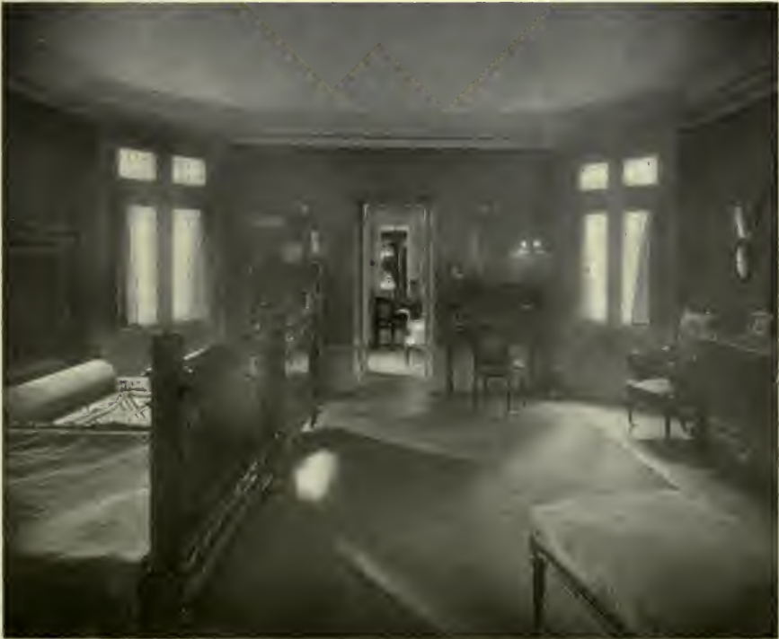
FIG. 7.—BEDROOMS IN THE HOUSE OF MR. M. NEWBORG. No. 50 East 52d Street, New York City. J. H. Freedlander, Architect.
