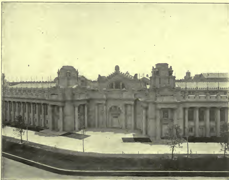
PROJECTING ANGLE OF THE ELECTRICITY BUILDING.
