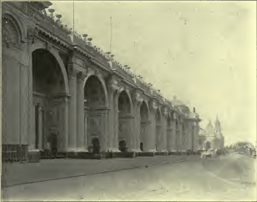
NORTH FAÇADE OF THE PALACE OF MANUFACTURES.
