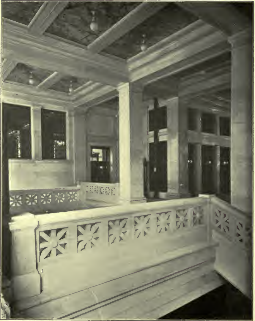
STAIRS AND HALL—FRICK BUILDING.
