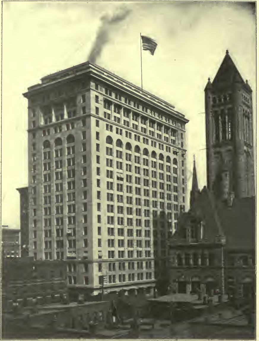
THE FRICK BUILDING.
