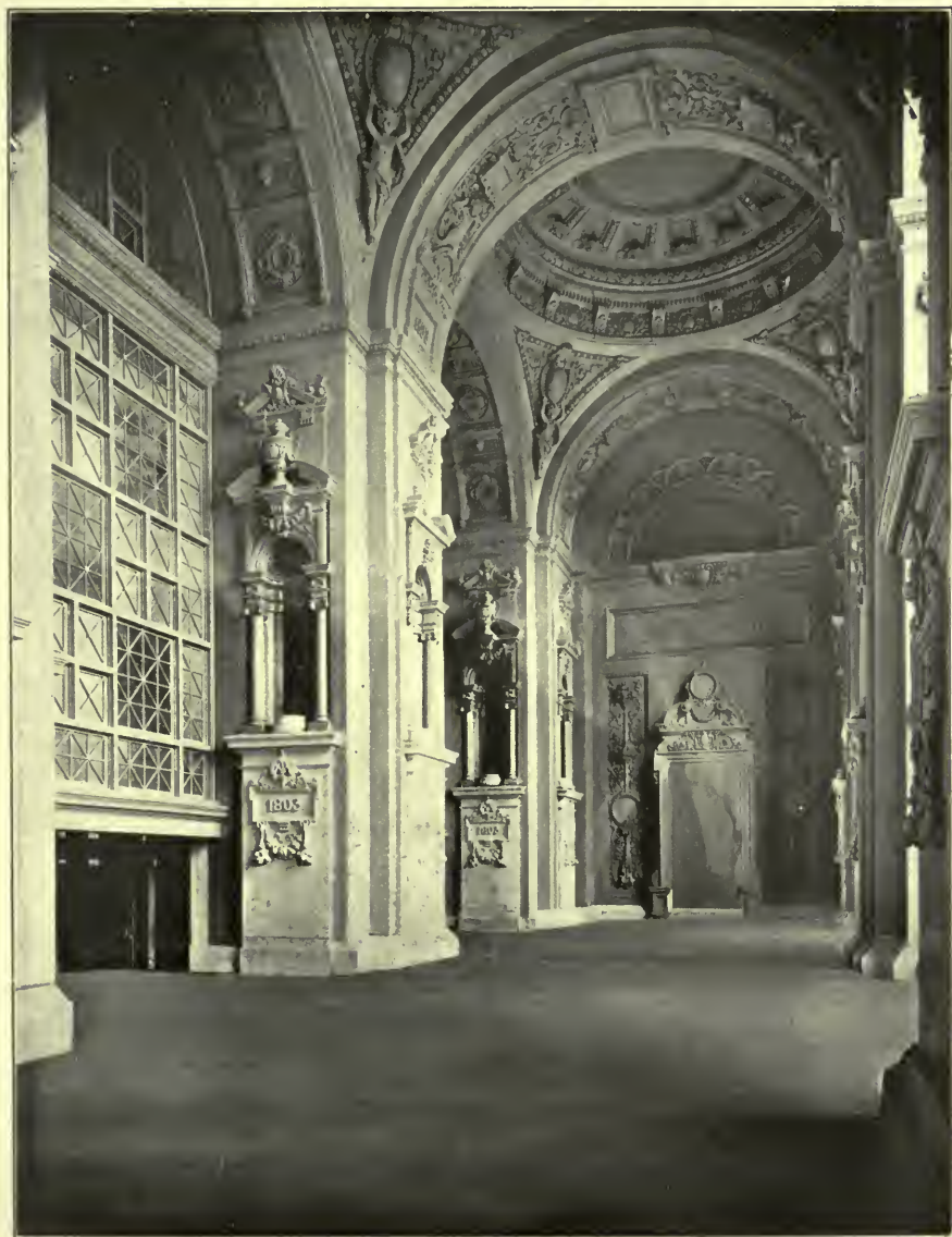
THE MANUFACTURERS' BUILDING—THE VESTIBULE.
