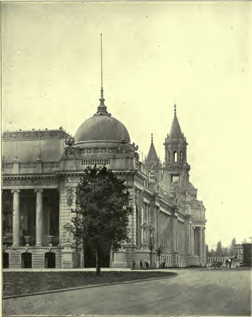
CORNER OF THE VARIOUS INDUSTRIES BUILDING.
