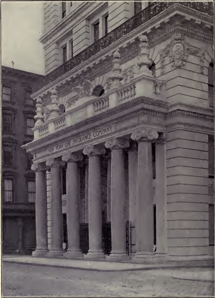
ENTRANCE, NEW YORK LIFE INSURANCE CO.'S BUILDING, Broadway and Leonard Street, New York City. McKim, Mead & White, Architects.
