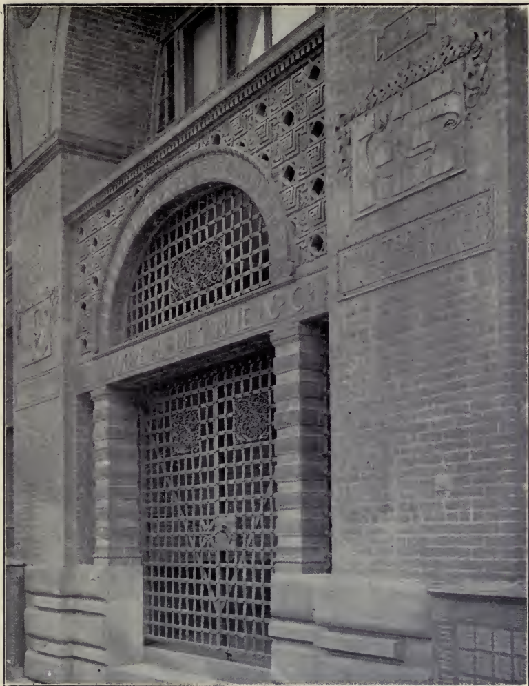
ENTRANCE TO THE DE VINNE BUILDING, Lafayette Place, New York City. Babb, Cook & Willard, Architects.
