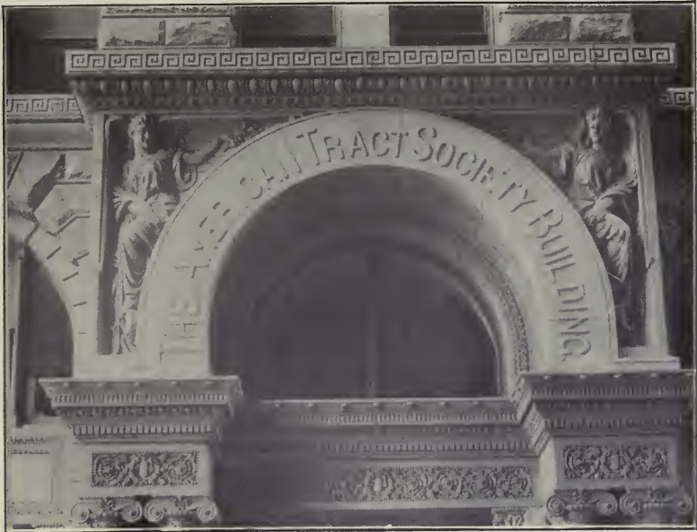
THE AMERICAN TRACT SOCIETY'S BUILDING. Nassau and Spruce Streets, New York City. R. H. Robertson, Architect.
